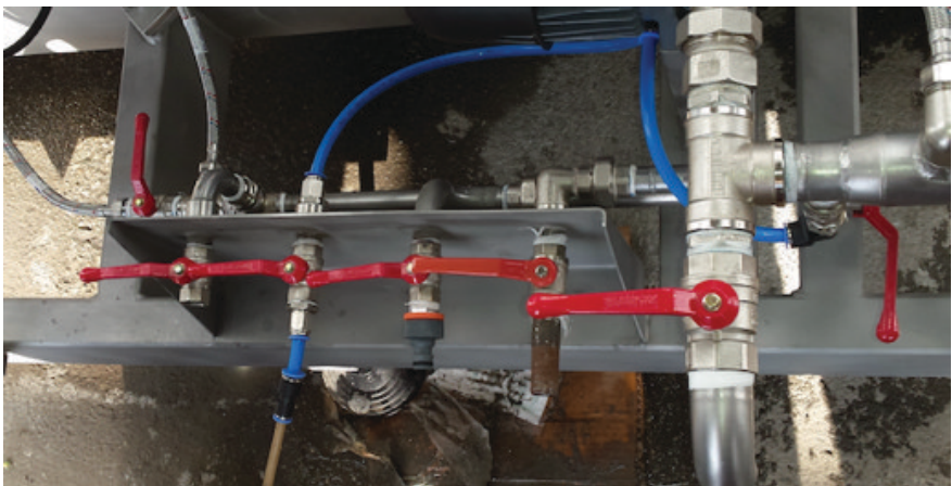
All connections to utilities at one spot.
